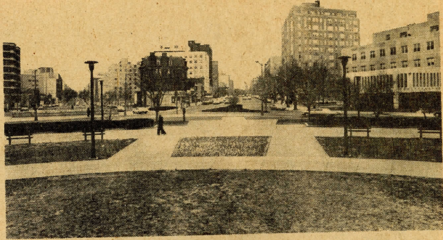
Washington Circle: facing east, the avenue to the left is "K" Street and the major thoroughfare to the right is Pennsylvania Avenue. The building to the extreme right is GW University Hospital.
